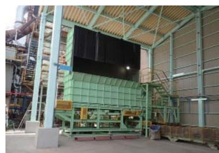
Shredded waste plastic hopper, extraction facilities (Kanda Cement Factory)
