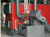
Biomass-fueled water boiler **Binder Boiler**
