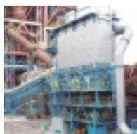
High-chlorine bypass facility at the Kanda Cement Factory
