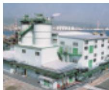
This plant turns incinerator ash into a raw material for cement.
