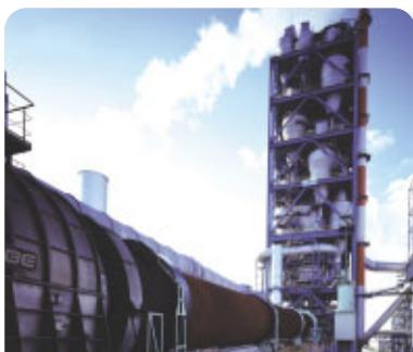
The new suspension preheater kiln at the Ube Cement Factory
